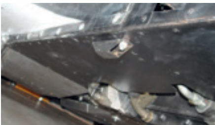
Lengthened engine bolts and 3/4" tube provide jacking points.
